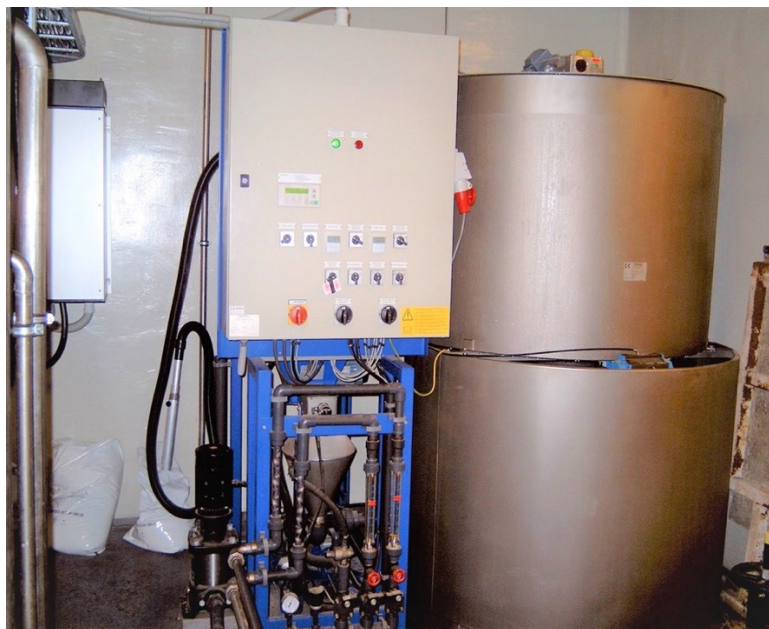
Figure 26. Polymeric Preparatory Unit for the WWTP of Liepāja city 21
