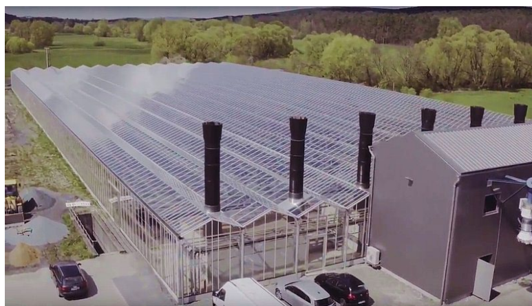
Figure 48. Covered fields for greenhouse sewage sludge drying 34
