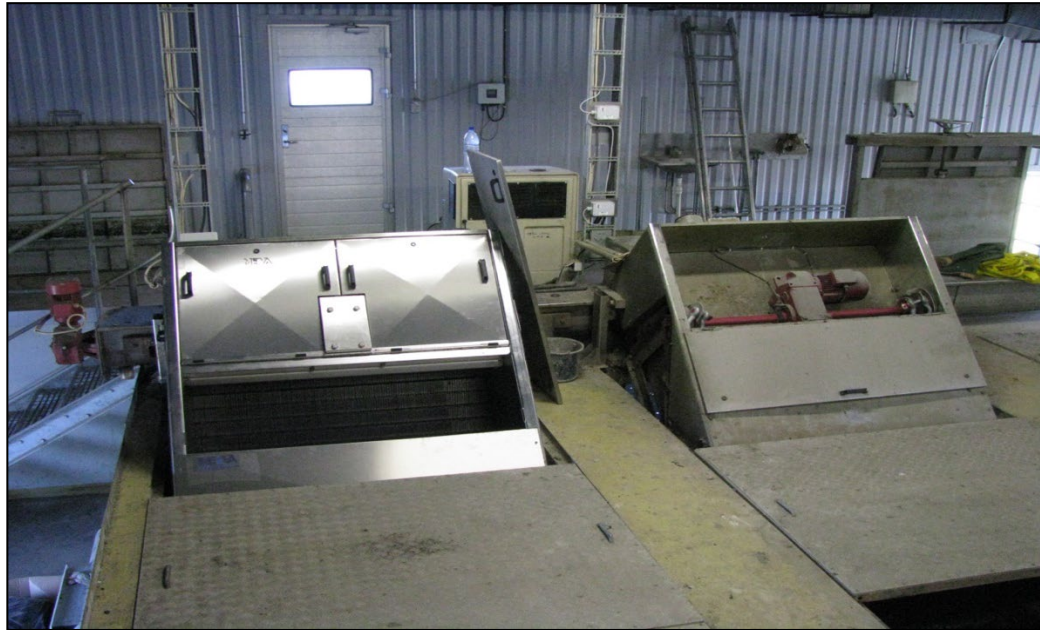
Figure 10. Mechanical bars at wastewater treatment plants in Liepāja, from “Liepāja Water” Ltd. archive
